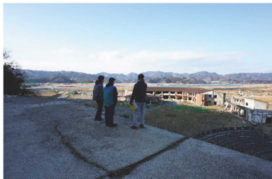
Fig.1 Disaster damage investigation
